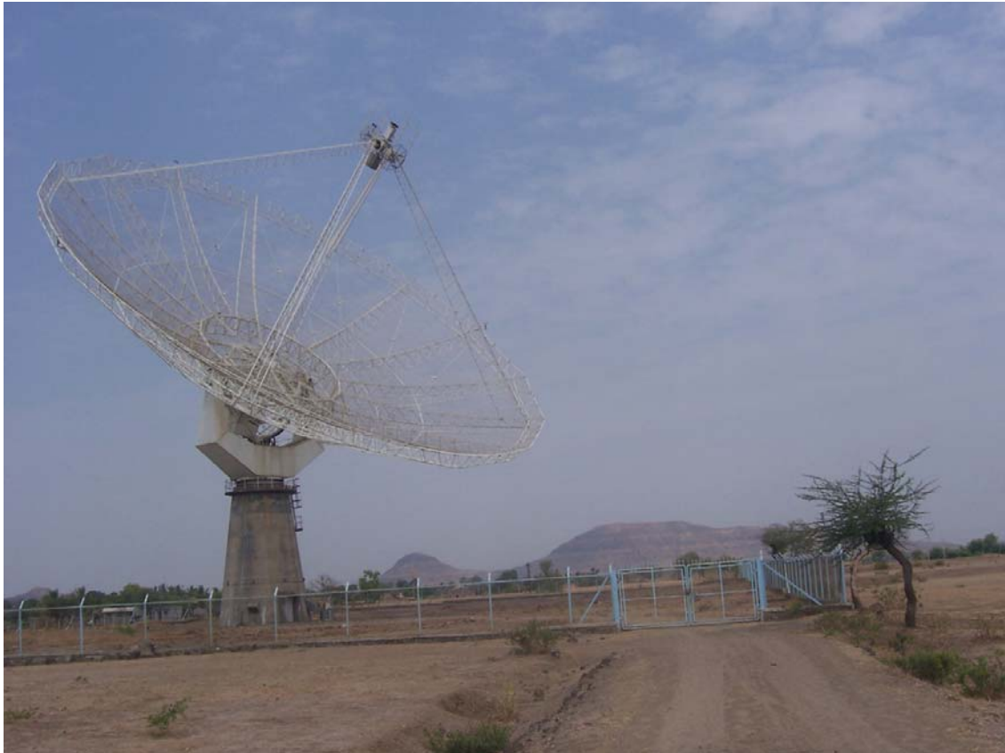
Fig shows one of the GMRT antennas
