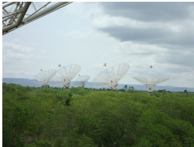
GMRT antenna array at center square.
