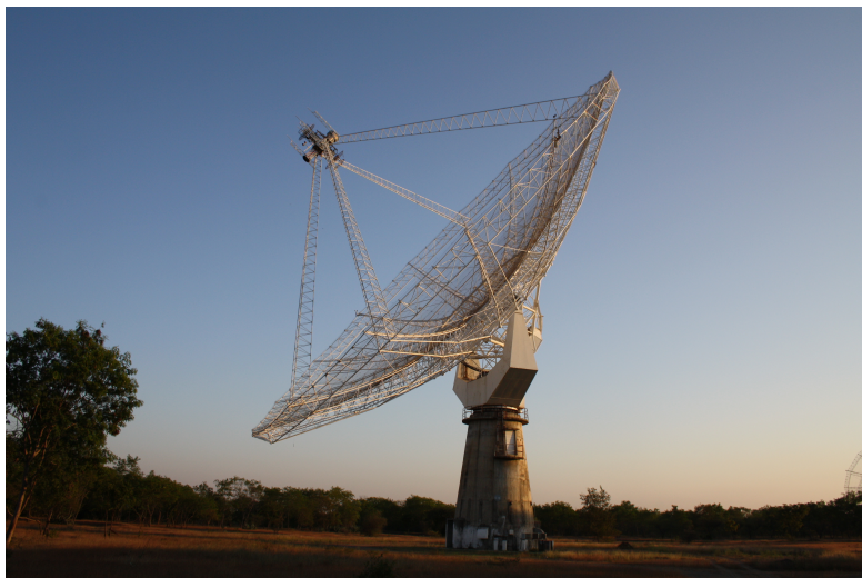
Figure 1.1: C8 Antenna at GMRT Central Square (Photo courtesy of Dipak Buch)
