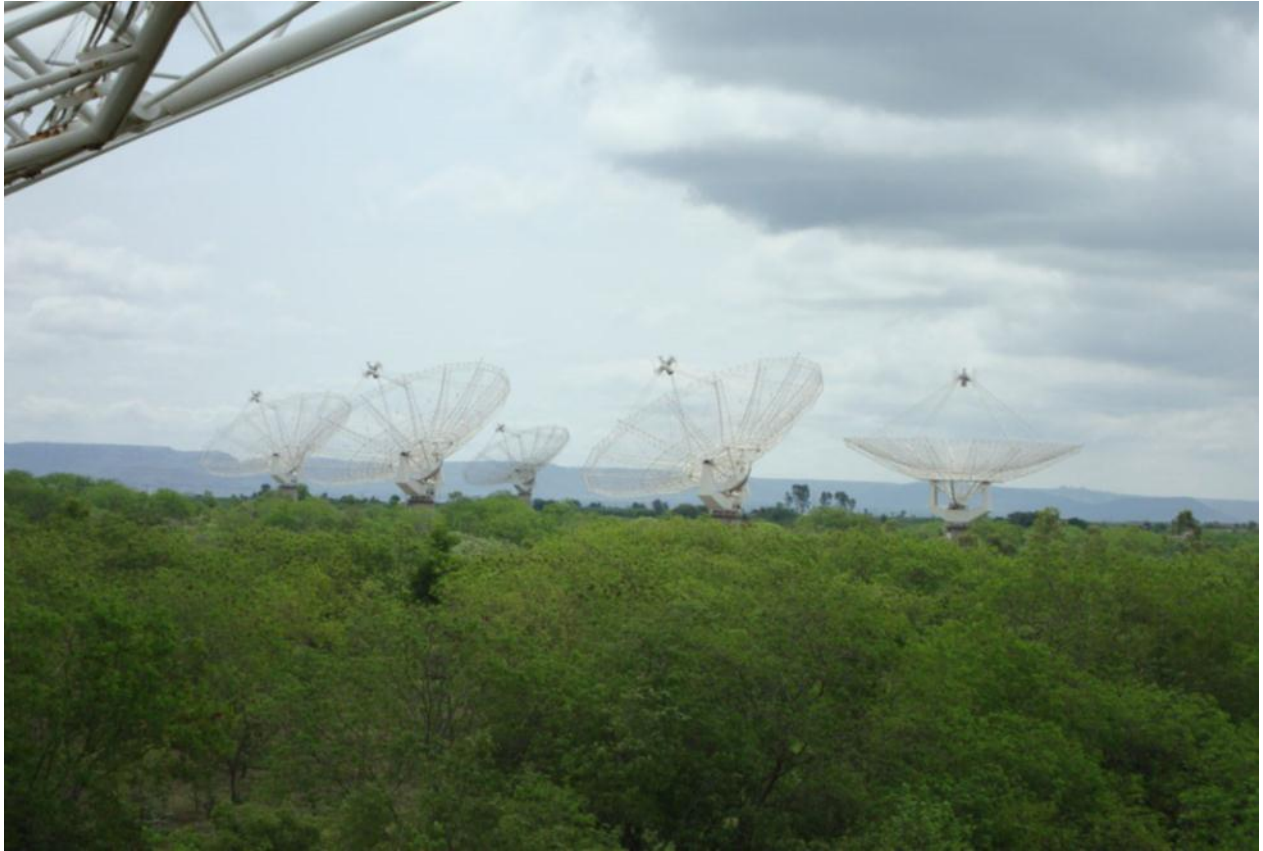
Figure 1-1 GMRT Antenna Array
