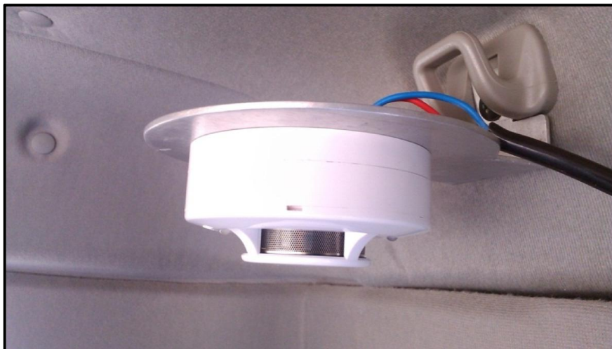
Fig. 9.3: Sensors installed in HLP.
