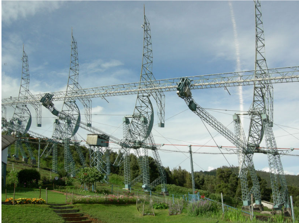
FIGURE 3.5: The Ooty Radio Telescope. The tall structure seen in this image is the metal frame supporting the dipoles as well as carrying the front end electronics for a single module. Photo credit: rac.ncra.tifr.res.in/rac_images/ORT02.jpg
