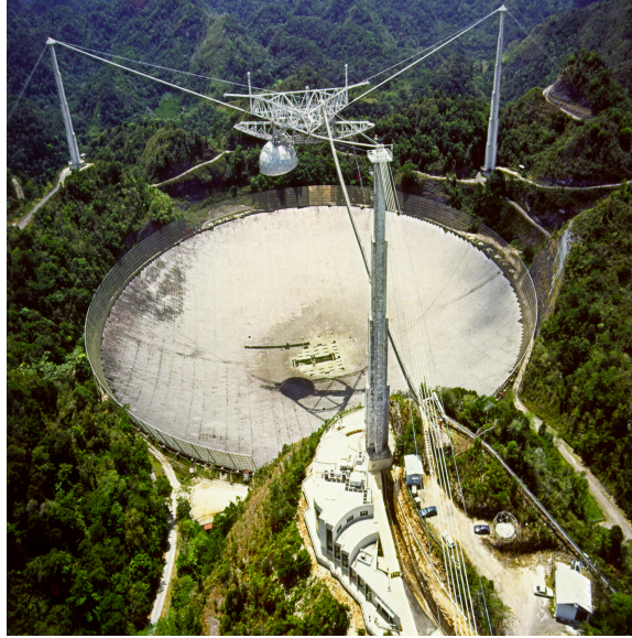
Figure 3.4. The Arecibo radio telescope solid dish. The feed is suspended above the fixed reflector by stretched cables from three supporting legs. It is located at 66^{\circ}45'10''\text{W} and 18^{\circ}20'39''\text{N} in the Puerto Rico, USA. (Credit : www.naic.edu )
