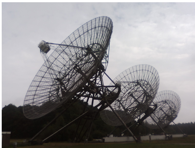
Figure 3.2. Three of the WSRT antennas. Last two antennas can be seen on the rail tracks. The WSRT is situated at 6^{\circ}36'15''\text{E} and 52^{\circ}55'00''\text{N} in the Netherlands.
