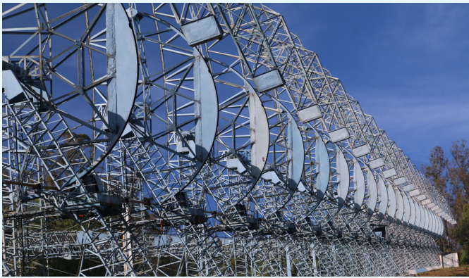
The ORT, a 530m long and 30m wide parabolic cylinder with its long axis parallel to that of the earth.
