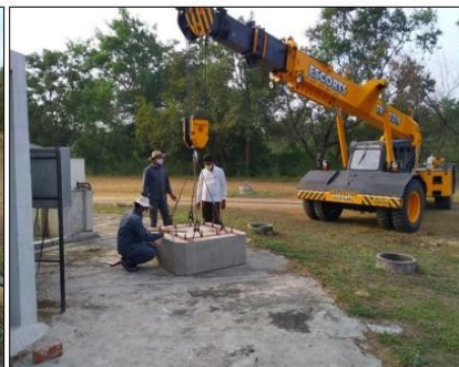
Concrete Block installation
