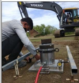
Plate Load test- soil Bearing Capacity
