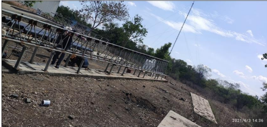
Quadripod legs Fabrication
