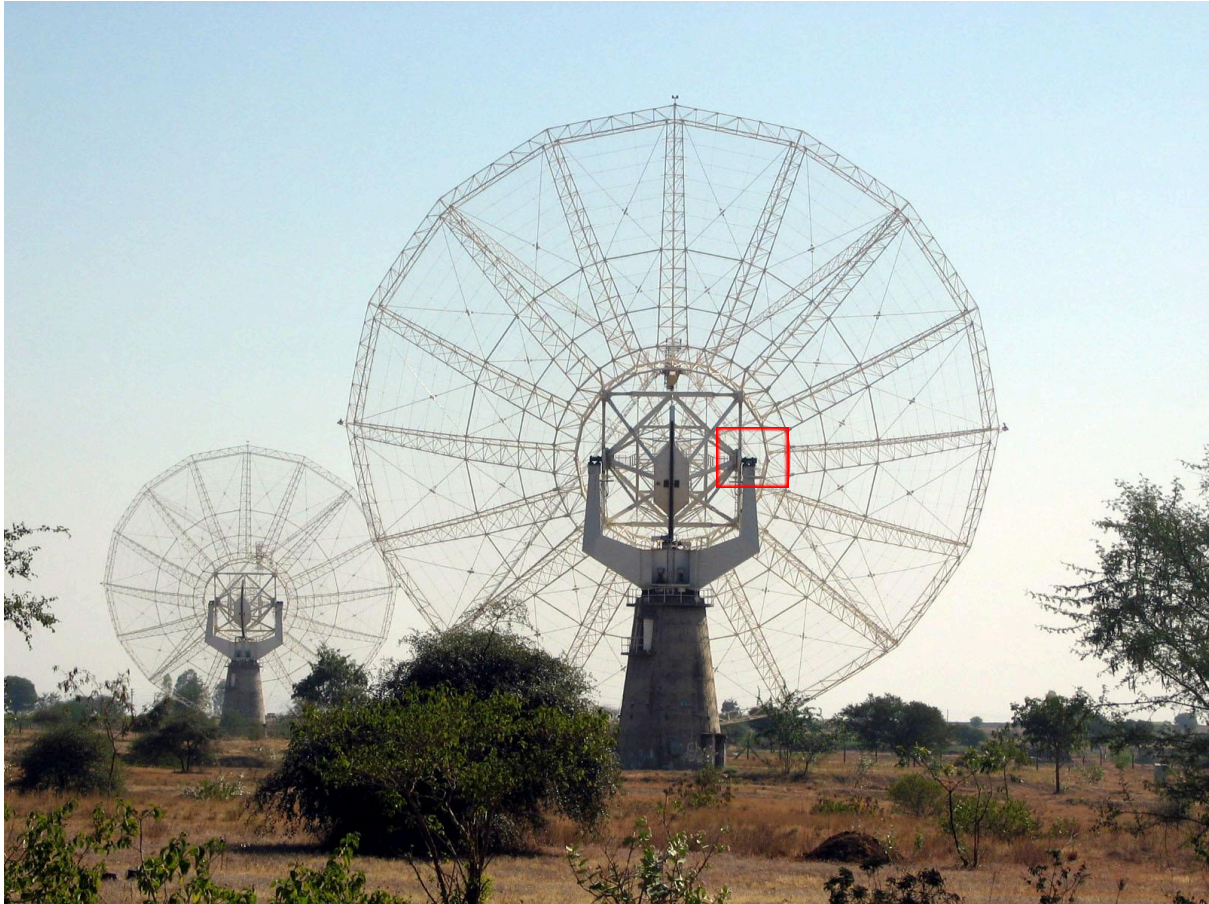
Fig 1. Red square box shows the EL axis encoder location
